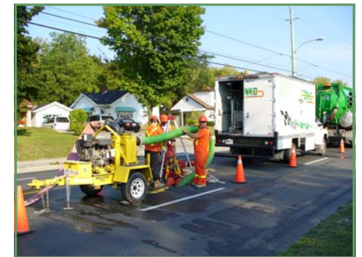
Bypass set-up by Benko to facilitate CCTV inspection and cleaning.
